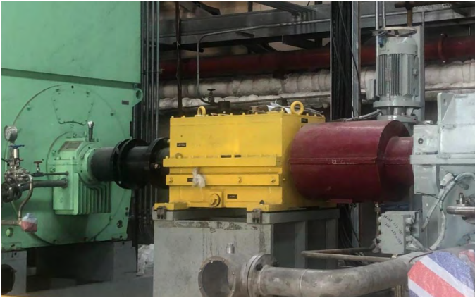
Housing Freewheel FHHS 18000 in water pump
